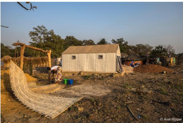
Set up of a Better Shelter kiosk, initiated by the IKEA Foundation. Two 70Kg-boxes, a manual and 6h of setting up.
